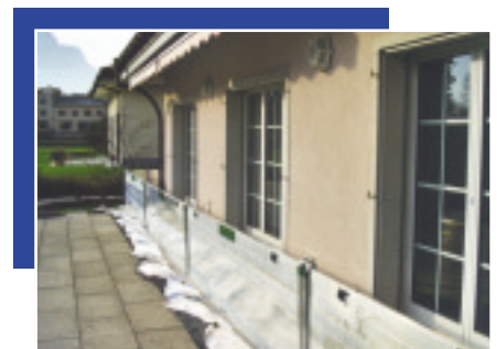
Sealing the shell of buildings (mobile)
