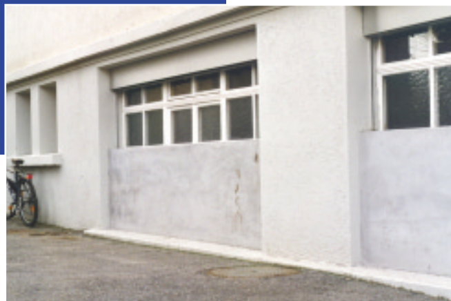
Sealing openings (permanently) by water resistant walls
