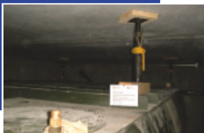
Oil tank protection against buoyancy (Basel)
