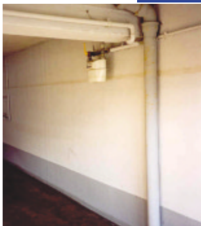
Elevated gas supply installation
