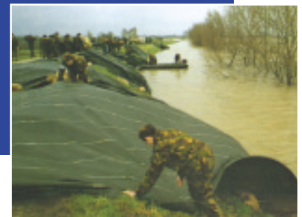
Flood fighting: shielding an embankment
