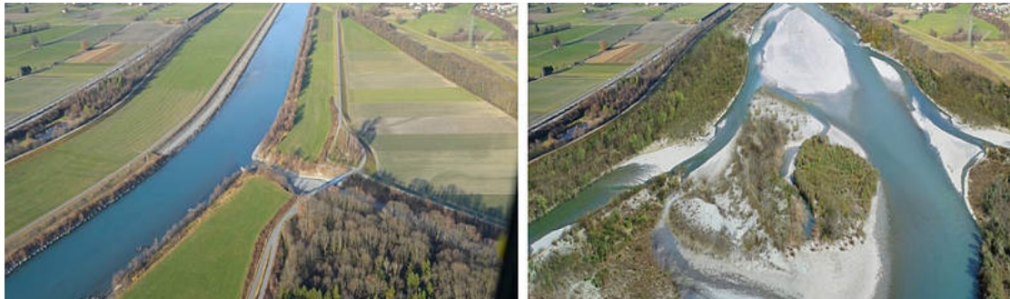
Figure 5a: Example of extension on the Alpine Rhine at the mouth of R. Frutz in Au, Vorarlberg, Austria (Source: Renaturierung Alpenrhein /©: Internationale Rheinregulierung IRR/Hydra-Institute, Peter Rey)
